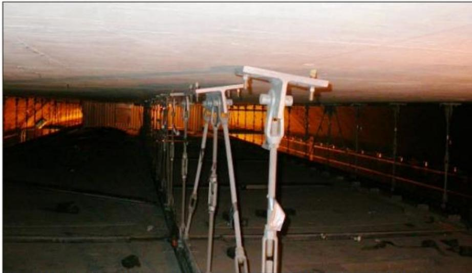
Figure 10. This photograph, taken in the westbound D Street portal tunnel after the accident, shows a number of roof hanger plates that have begun to pull away from the tunnel roof, including the two-anchor hanger plate in the foreground and the four-anchor plate adjacent to it.
